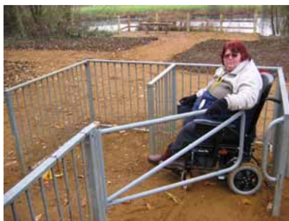
The original kissing gate proved adequate for wheelchair access but unsuitable for use by powered chairs
